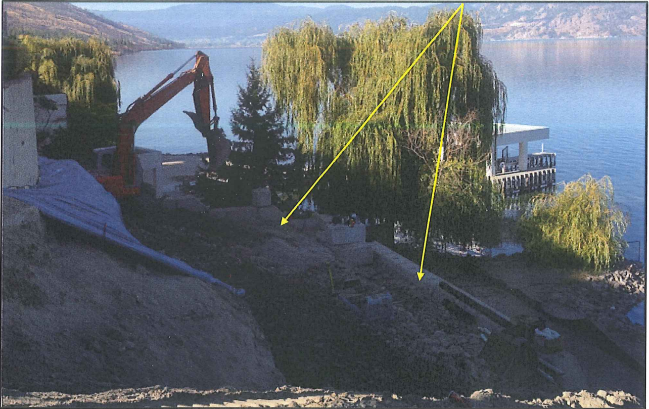
Photo 2: Foreshore Reconstruction and Over-height Lock Block Retaining Walls (from above)
